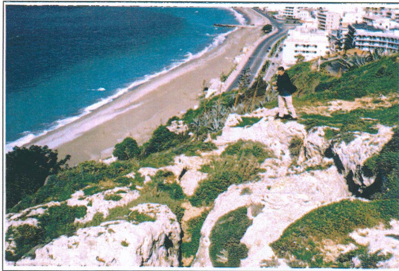
Figure 4: Boulders that can block the road, which links the town with the airport, in the case of earthquake.
