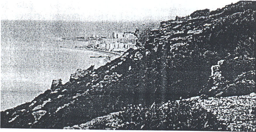
Figure 6: Demolition of the unstable rock boulders at the Monte Smith hill.
