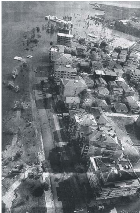
Figure 7: Subsidence at the coastal zone of Gölçük. The location is within a pull-apart basin created by the distribution of strike-slip movement.
