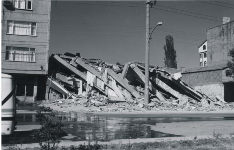
Figure 9: Collapsed multi-story buildings, lying close to the seismic fault. Eastward and westward card-deck collapse is indicative of large surficial displacement, a fact confirmed by instrumental recordings.
