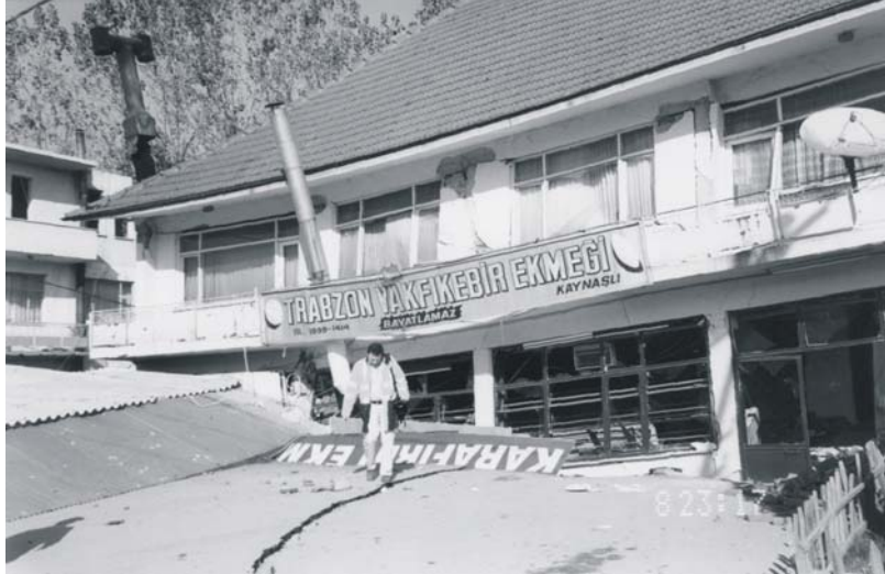
Figure 8: A construction with R/C frame, sunk into the loose surficial formations within a flower structure.
