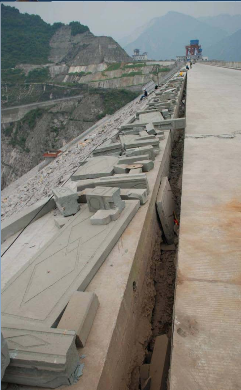
Fig. 1 Sliding failure of an earth dam
